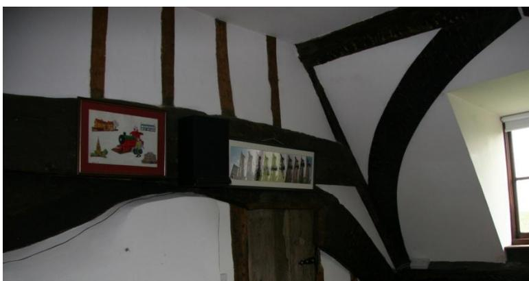
Figure 4: The arch of an open-hall truss, visible in the attic.
