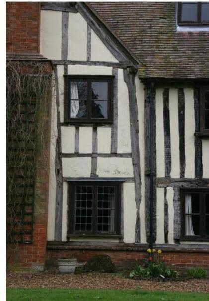
Figure 6: The second medieval hall (left) and (right centre) the corner posts of the two frames, side-by-side.
