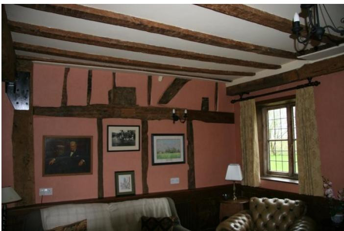
Figure 10: Oak framing inside the 'solar'
